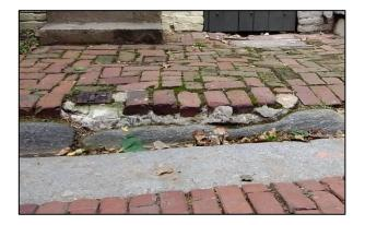
**Image 6:** Severely eroded curb stones along parking area, northwest end of street
