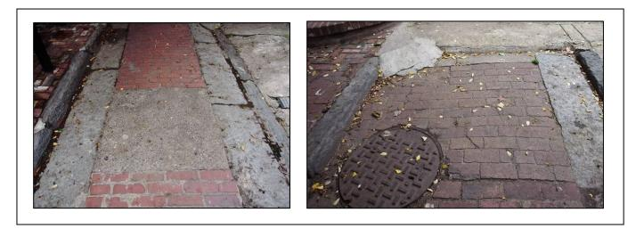
**Image 13:** Left: section at south end of South Jessup Street which has been repaved with concrete. Right: section at south end of South Jessup Street which has been repaved with contemporary brick.
