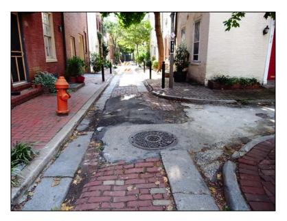
**Image 12:** Intersection of South Jessup and Latimer Streets where original paving materials have been removed/paved over
