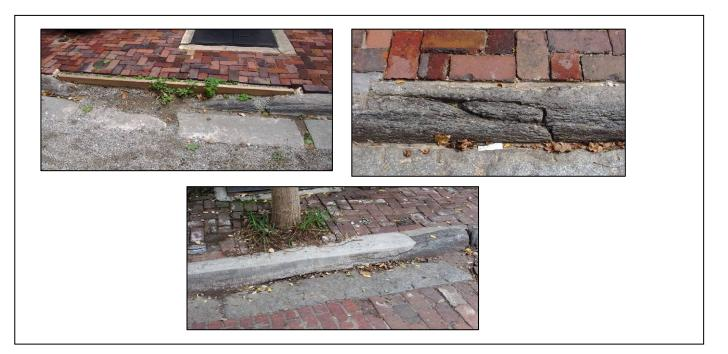
Image 8: Clockwise from left: sunken curb stone, cracked curb stone and curb stone partially covered by cement
