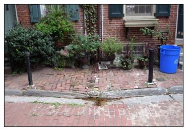
**Image 16:** Section of sunken paving between houses 227 and 229
