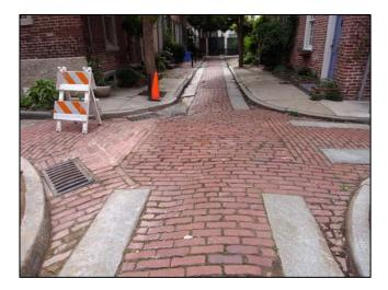
**Image 15:** Section of uneven paving at the intersection of South Jessup and Irving Streets
