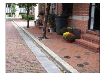
Image 4: Concrete replacement curb, northeast end of street
