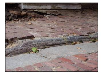
**Image 9:** Abrasions on surface of curb stone due to municipal snow removal equipment
