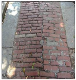
**Image 14:** Section of replacement brick which includes mismatched brick and brick fragments
